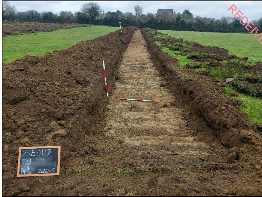
Plate 13 Trench 9 looking north-north-east
